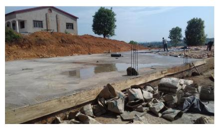
The slab has to be built right, because its state affects every other wall that will be raised on it. It has be built to bear the tonnage of focused-weight. So each part is built to bear that pressure.
