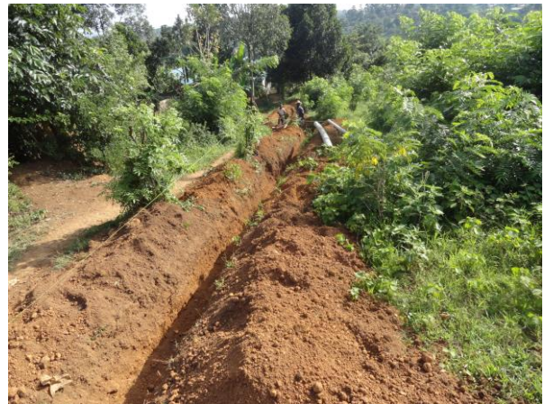
Drainage to the septic tank and soak pit
