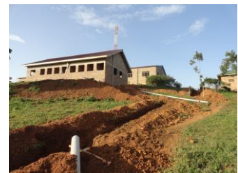
Drainage to the septic tank and soak pit
