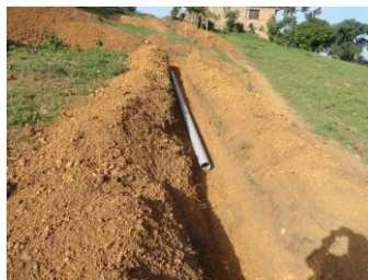
Drainage to the septic tank and soak pit
